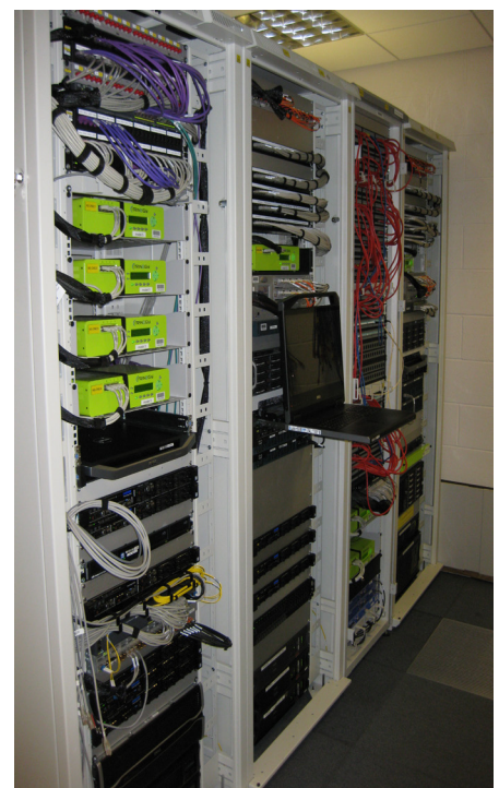
NE-ONE Professional and NE-ONE Enterprise Network Emulators (green appliances) are an integral part of LSRC's test set-up
