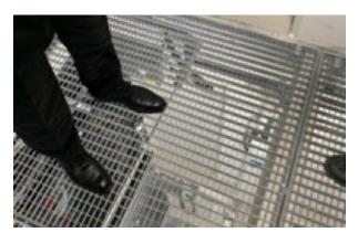
Each floor of the five-story Marilyn Datacenter is partitioned, structured in hot and cold aisles. The cooling mode in free cooling involves circulation of outside air, made possible by separations between floors by gratings and thus the absence of false floors, which are often source of problems in traditional data centers.
